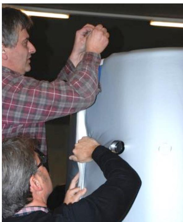
**NOTE:** Insert the insulation over sockets 1 – 3, hold it in place, and press it down firmly onto the buffer tank. Subsequently, pull the insulation tightly around the buffer tank. It is important to ensure that there are no gaps between the insulation and the buffer tank. If necessary, press and tap on the insulation with a flat palm and pull it tight.
